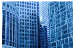
Structural Health Monitoring
